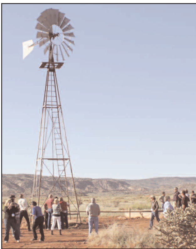
Tour members view the hand constructed tower of the windmill that pumps water for the cattle on the ranch. The ranch has one hundred such windmills on the land.
