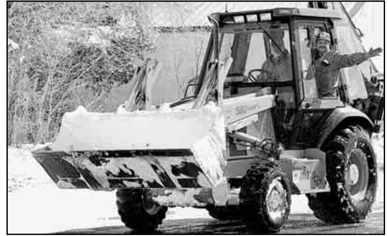
Baca Valley Telephone contributed crews and equipment Saturday to help Des Moines dig out.
