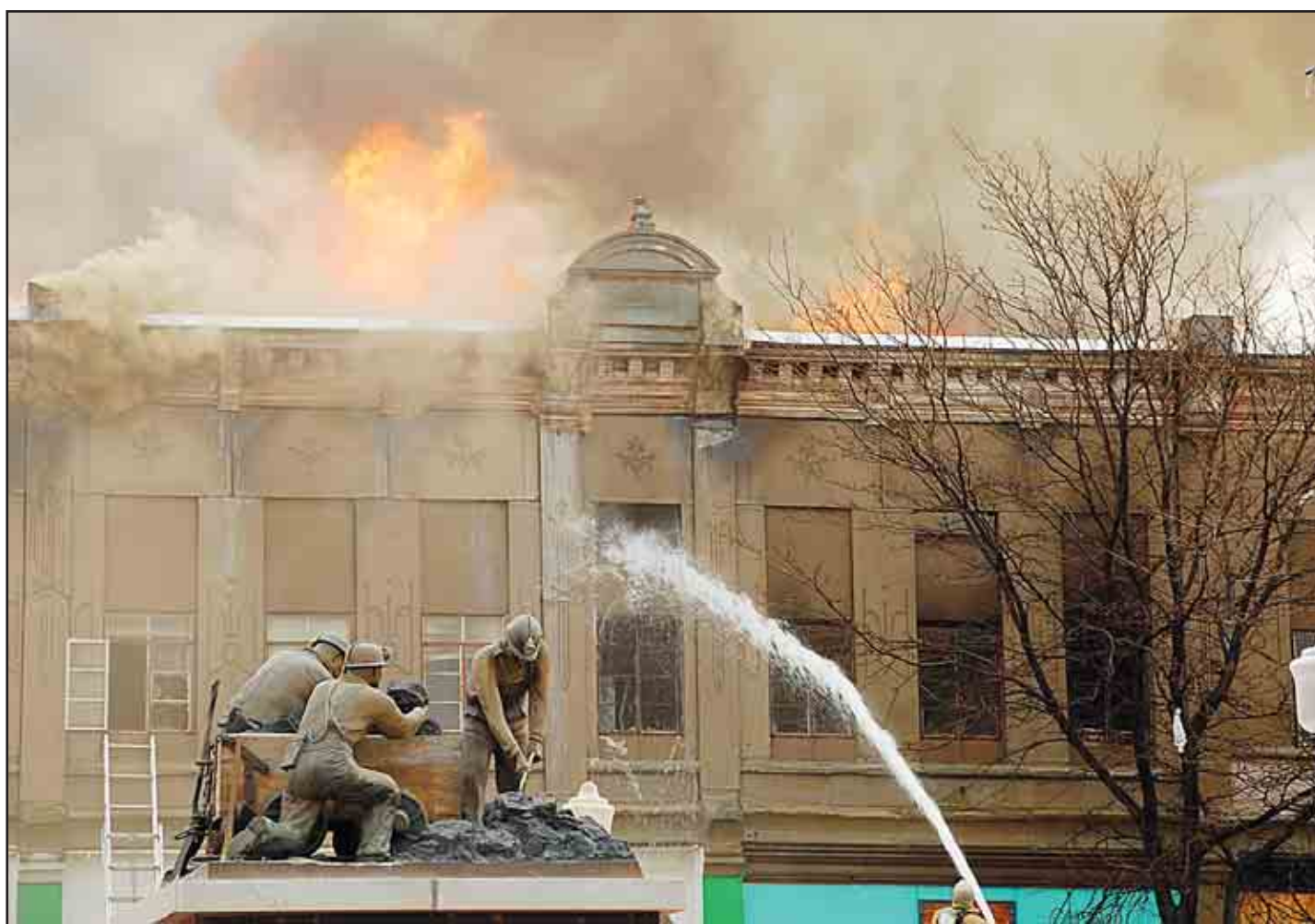
The Trinidad Fire Department battled the fire at the historic Franch building on Main Street until 10 p.m. on Saturday. The apartments on the second floor of the building were destroyed. The cause of the fire remains under investigation.
